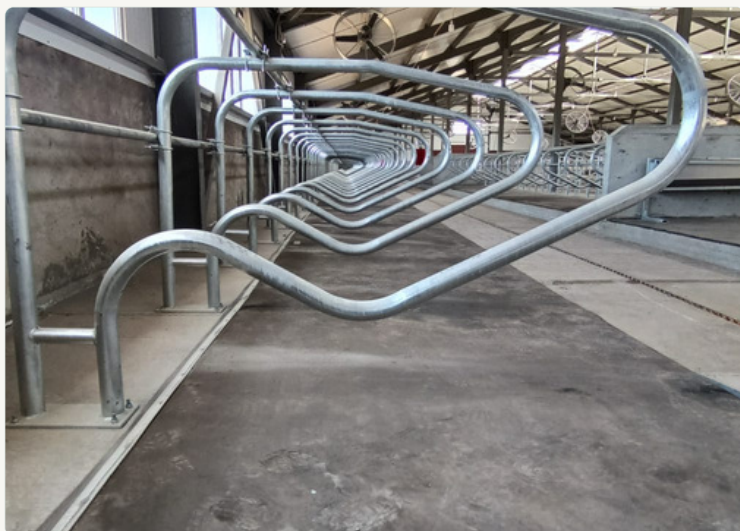
Cubicle division arrangement / Cubicle installation inside the barn
