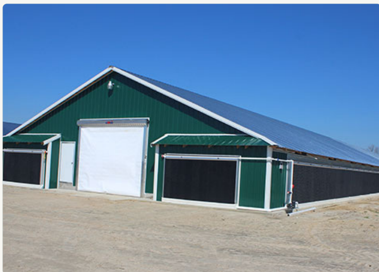
Barn cooling installation / Evaporative media detail
