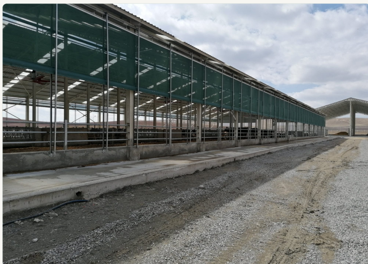
Barn side-curtain installation / Closed curtain arrangement
