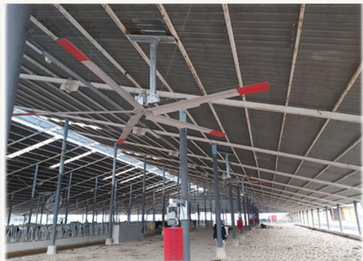
Ceiling-fan installation / Circular-fan installation
