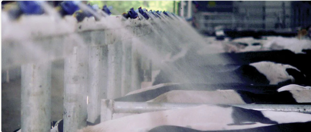
Sprinkler line over the occupied area
